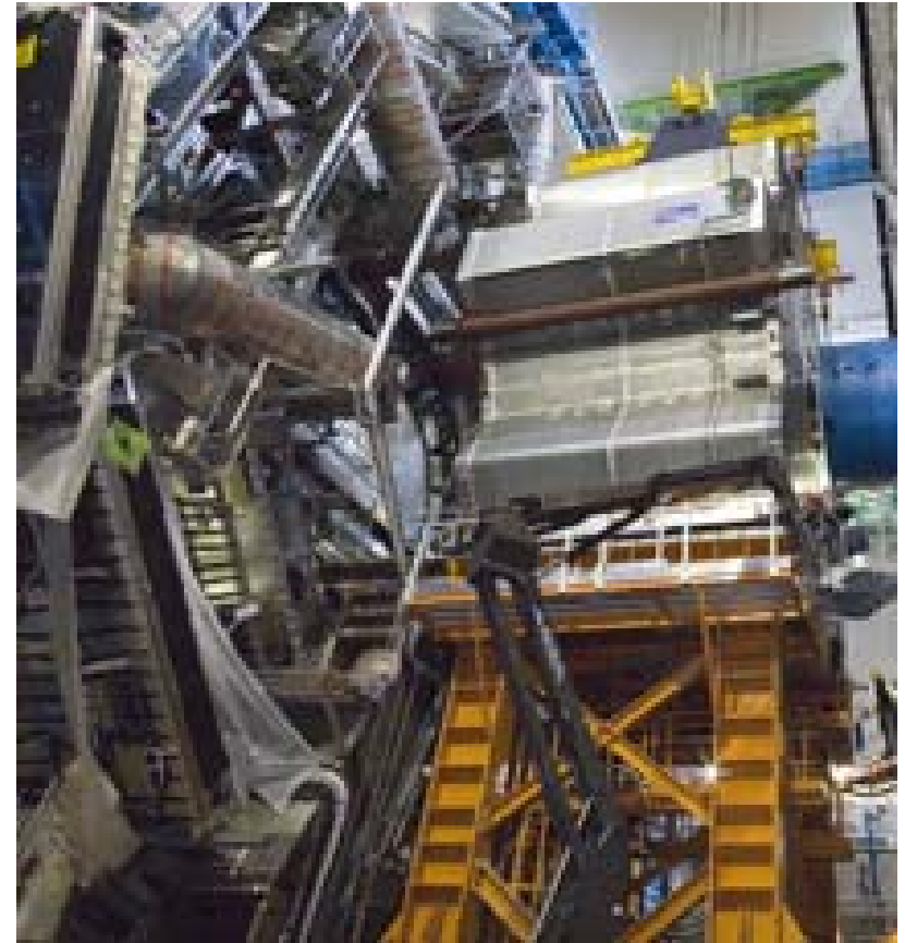
End-Cap Toroid A after lowering into the cavern on 13 th June 2007
